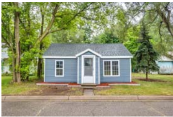
This home is stick built on a foundation and measures 558 square feet
