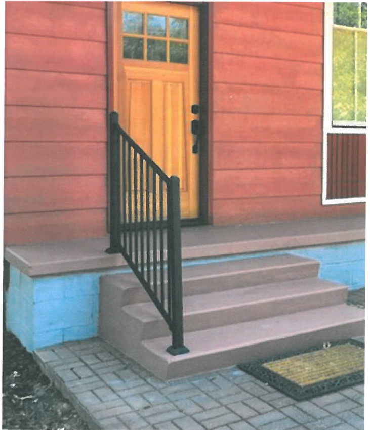
Studio Stairs After
