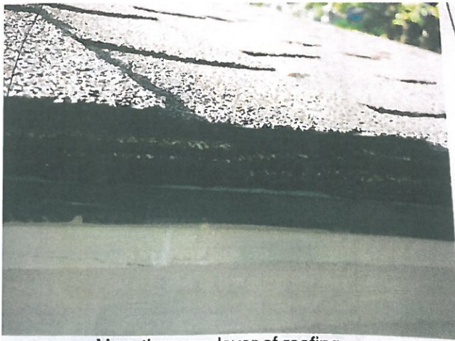
More than one layer of roofing
