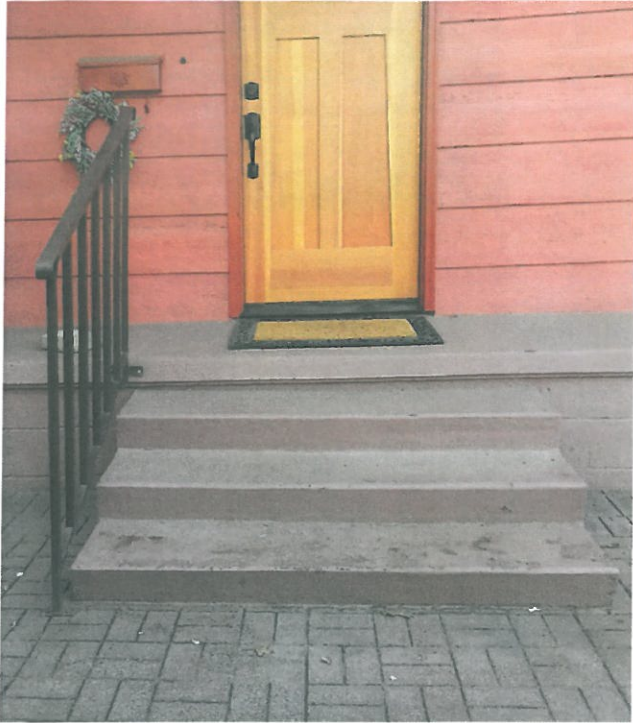
Main Stairs Before
