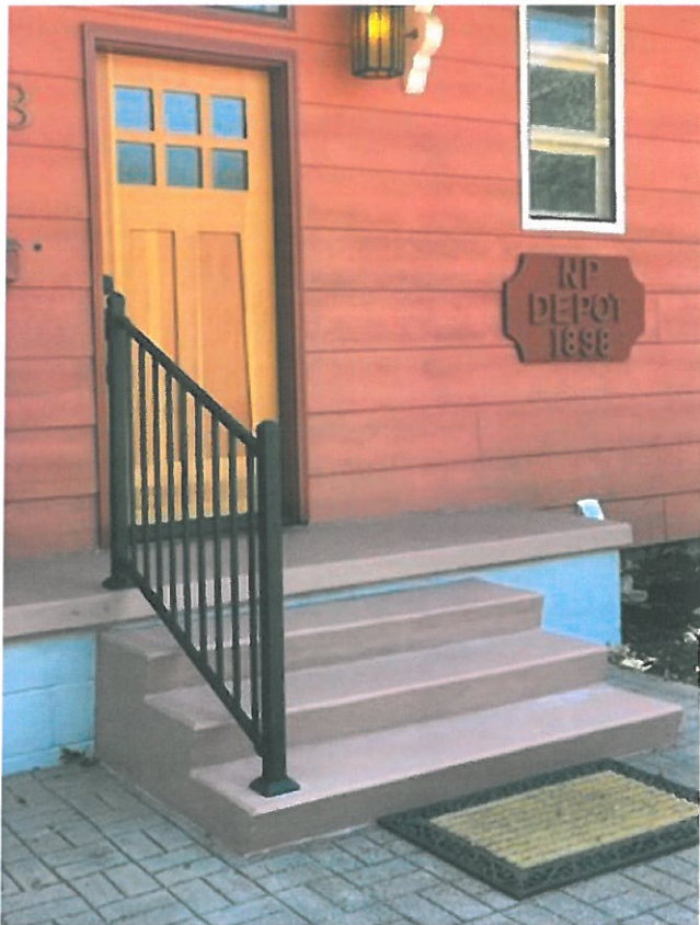
Main Stairs After
