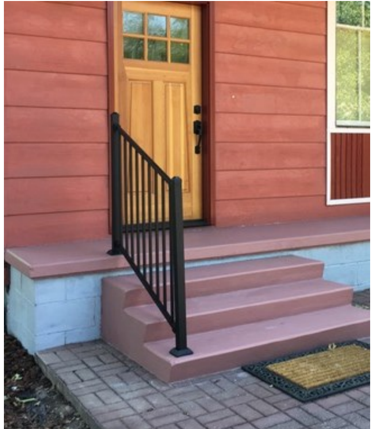
Studio Stairs After
