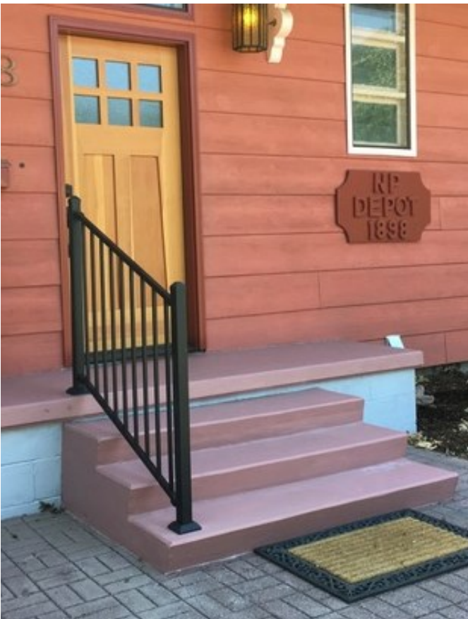
Main Stairs After
