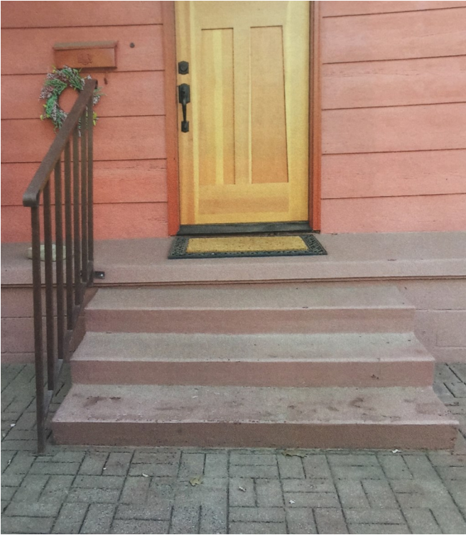
Main Stairs Before
